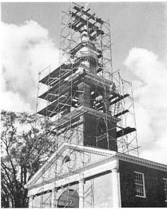
FIG. 5. Lebanon Meetinghouse. Rebuilding the spire.
