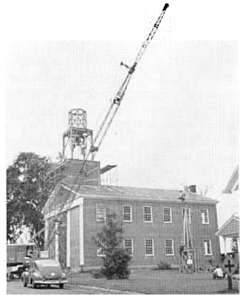
FIG. 4. Lebanon Meetinghouse. Rebuilding the spire.
