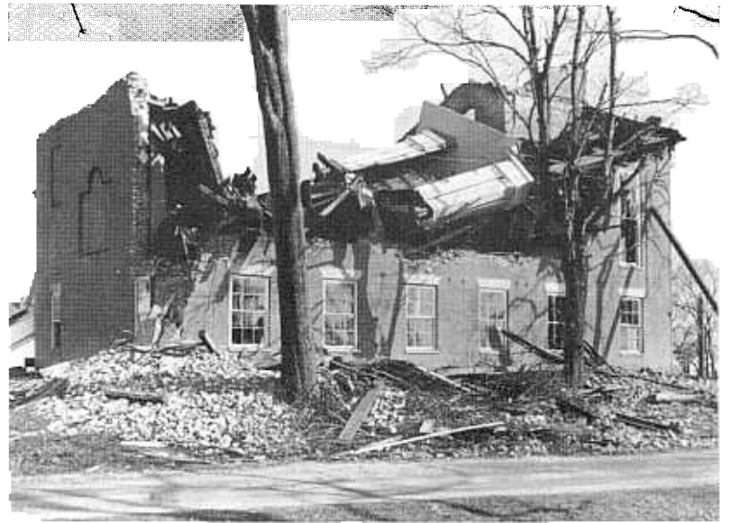
FIG. 2. Lebanon Meetinghouse after the hurricane of September 1938.
