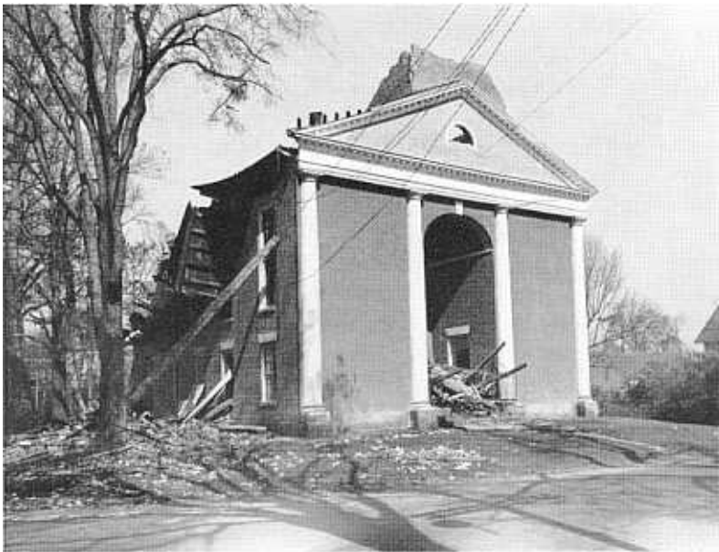
FIG. 3. Lebanon Meetinghouse after the hurricane of September 1938.
